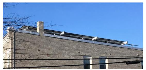
In other instances, the panels can be mounted directly to the roof surface, although articles noted care has to be taken to not compromise the integrity of the roof.
